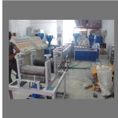
LDPE & PVC Kisan Pipe Plant
